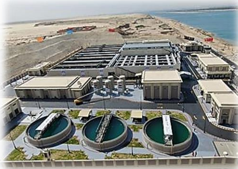
Bahr Al-Baqar tertiary treatment plant
